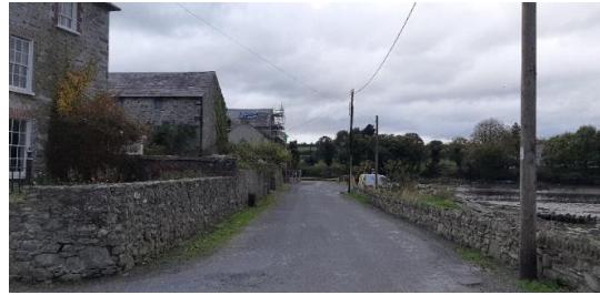
Image 6: View of Quays at eastern edge of site
